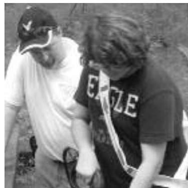
Mr. Barry and Todd Rowland power wash OA bridge
